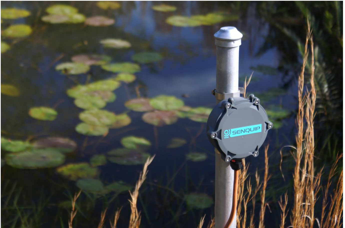
Figure 1 Battery Powered ORB-X1-G Monitoring Water Level
