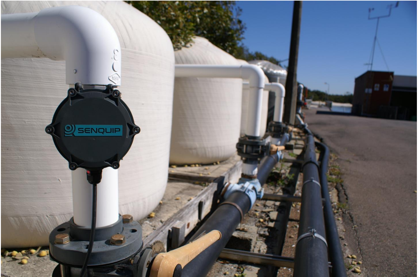
Figure 2 Battery Powered ORB-X1-W Monitoring Filter Pressure
